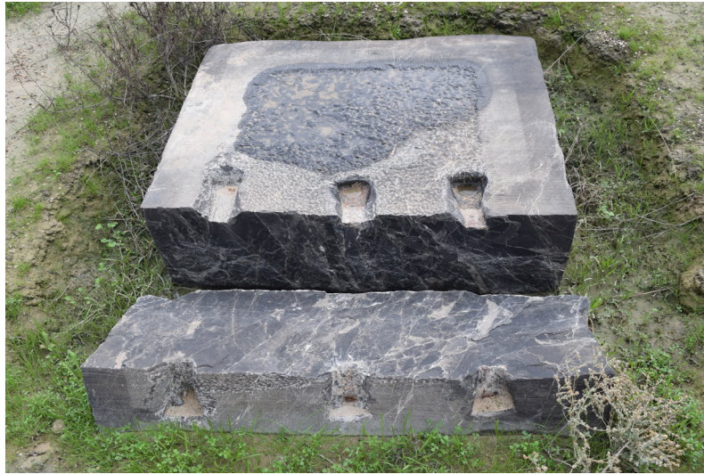
Fig. 48. Sang-e Siah: cavities indicating dove-tail clamps were used in the column base (photo by the author, 2018).
